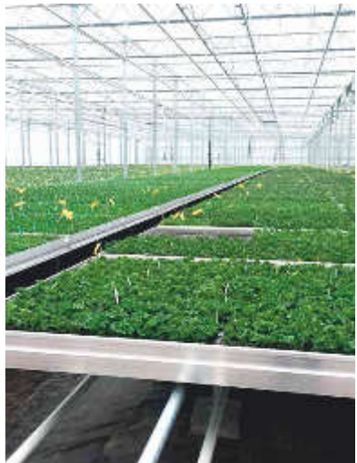
New Toscana rooting station facility.
